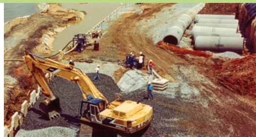
The above images show the construction of the Combined Sewer Treatment System that lies below the Riverwalk. Some of these lines are as large as 96 inches in diameter.
