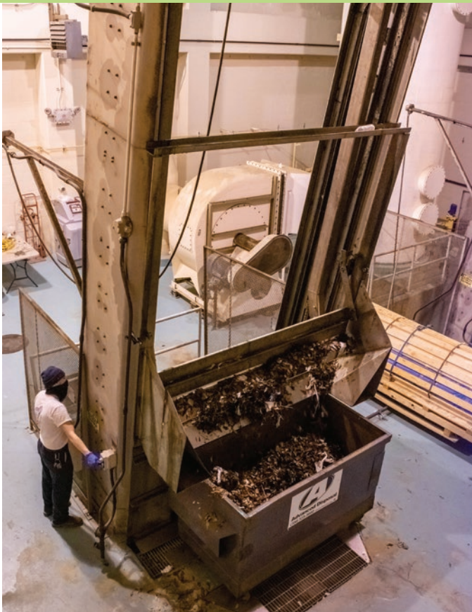
Technician cleans automatic bar screens which remove trash and debris from combined sewer lines to prevent it from going into the river.
