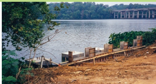
The above images show the construction of the Combined Sewer Treatment System that lies below the Riverwalk. Some of these lines are as large as 96 inches in diameter.
