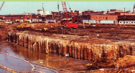
The above images show the construction of the Combined Sewer Treatment System that lies below the Riverwalk. Some of these lines are as large as 96 inches in diameter.
