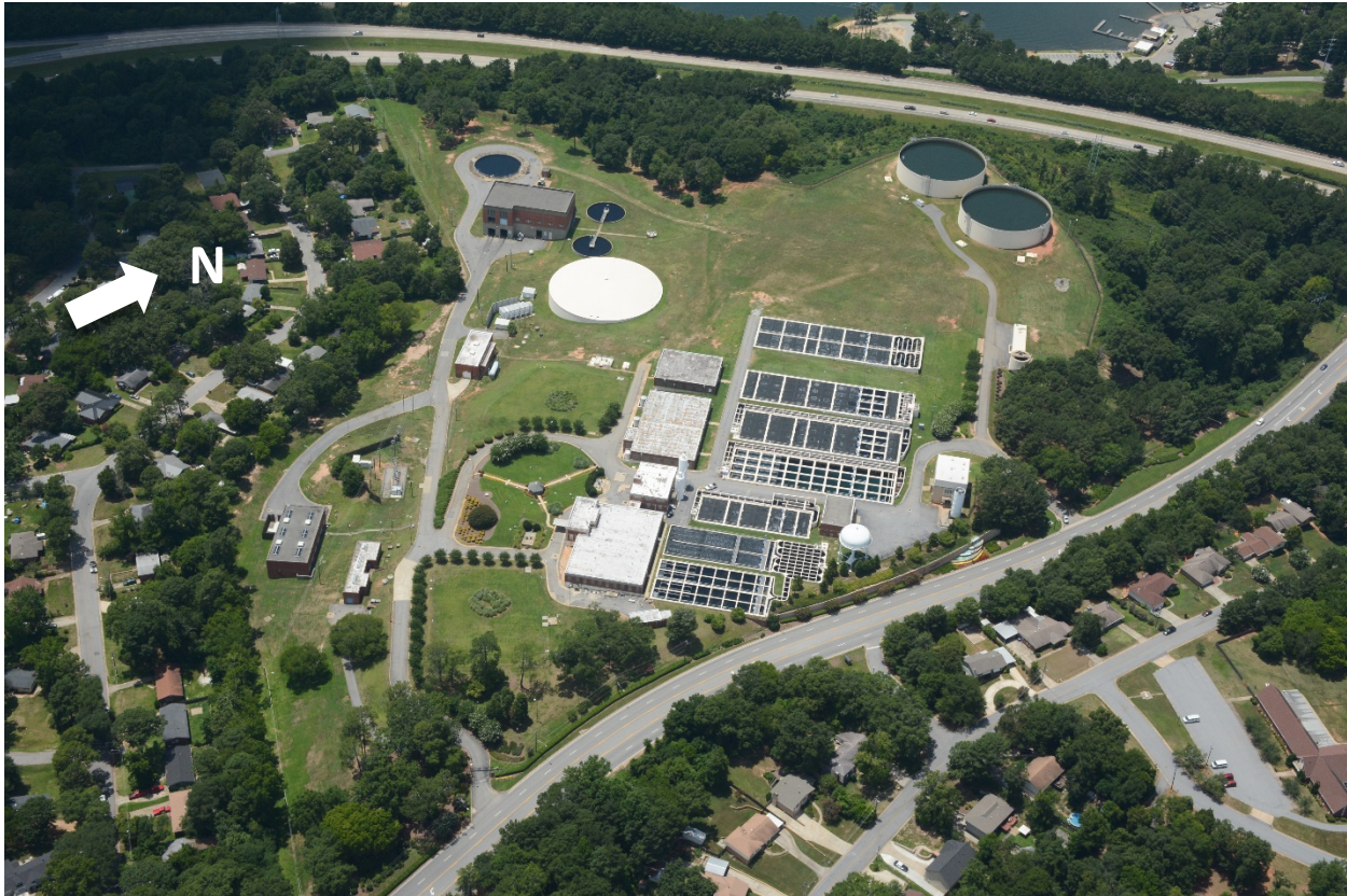
Figure 2.1 Aerial View of the NCWRF
